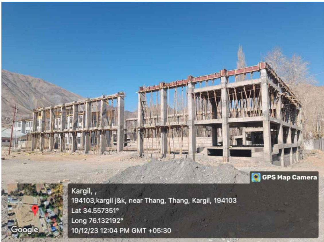
Under-construction of Indoor Stadium-cum-Multipurpose Hall
